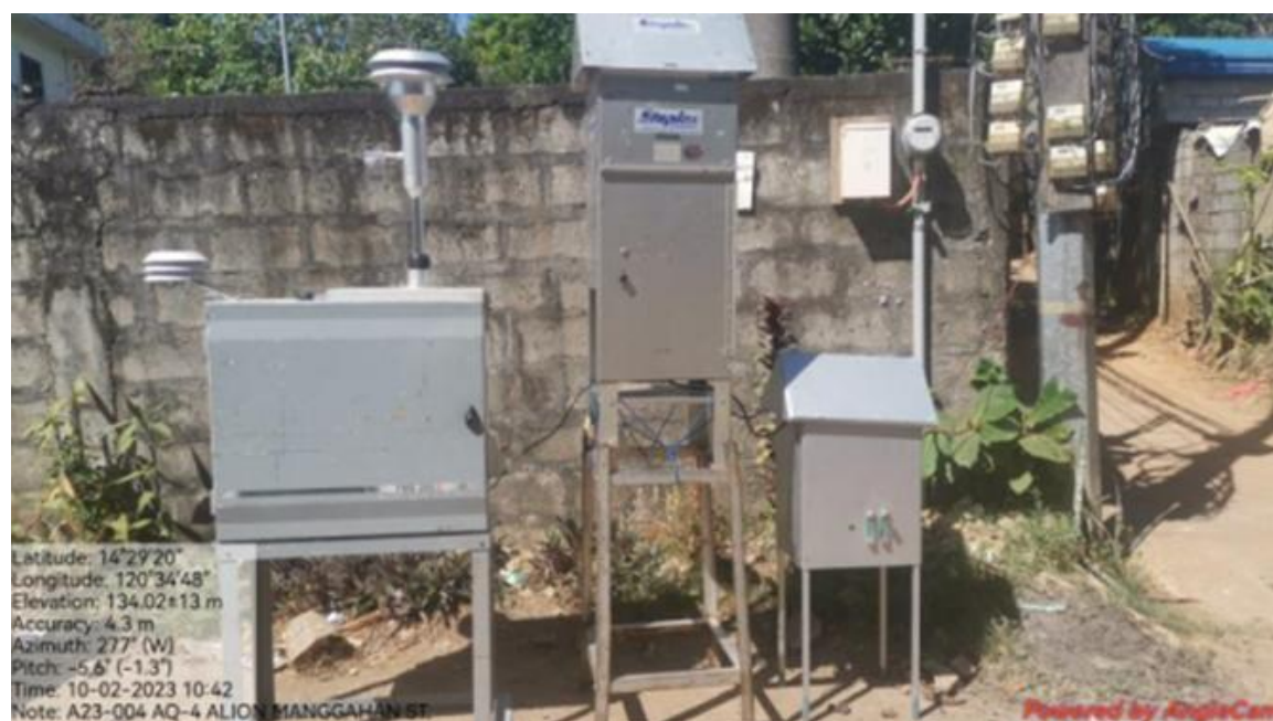
Plate 2- 34 Air quality monitoring at Station AQ4 in February 2023
