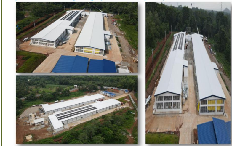
Fully Enclosed Building Design (Tunnel Vent System)
